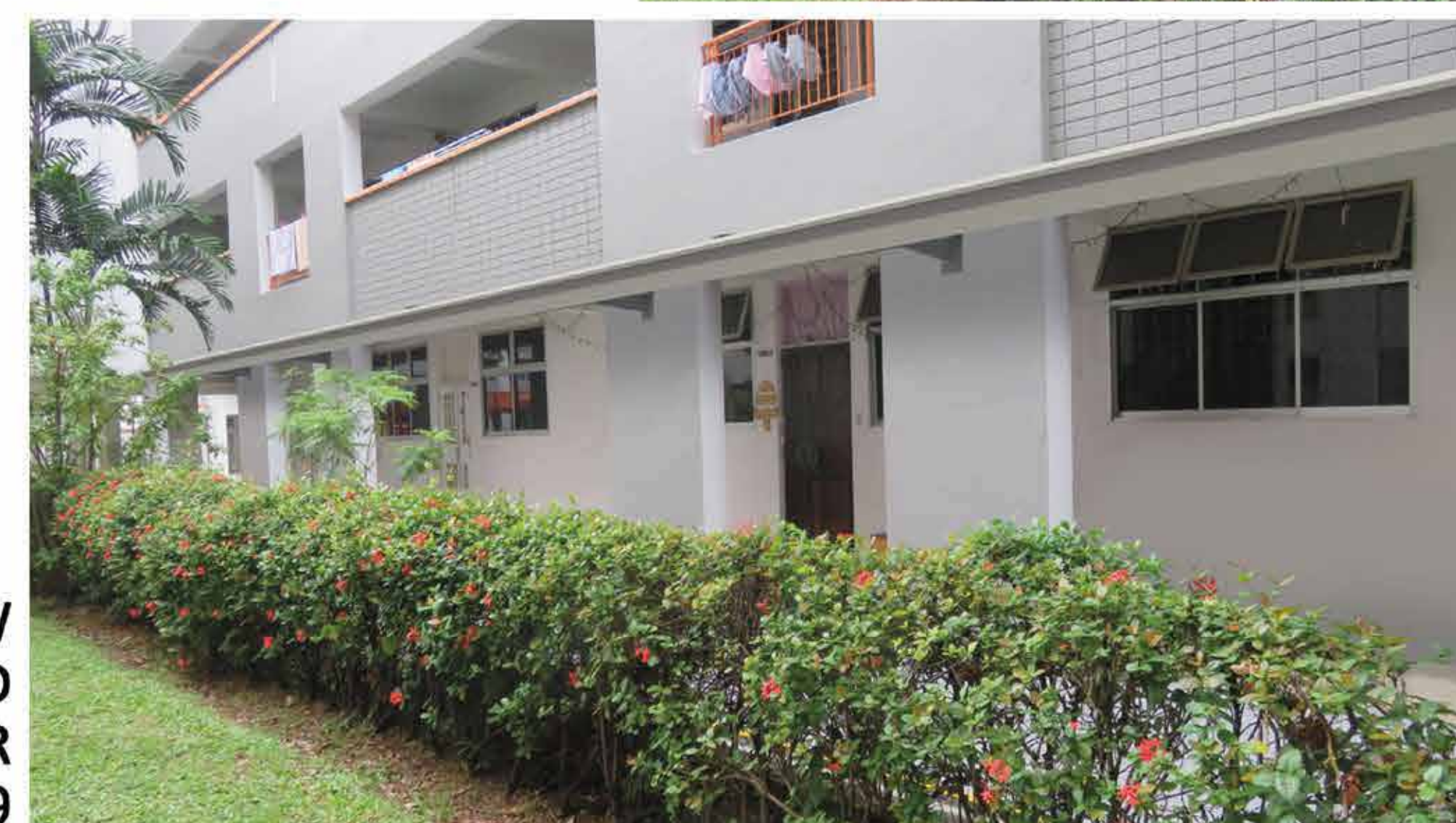
EXTERNAL VIEW OF EXTENDED CORRIDOR AT BLK 359
