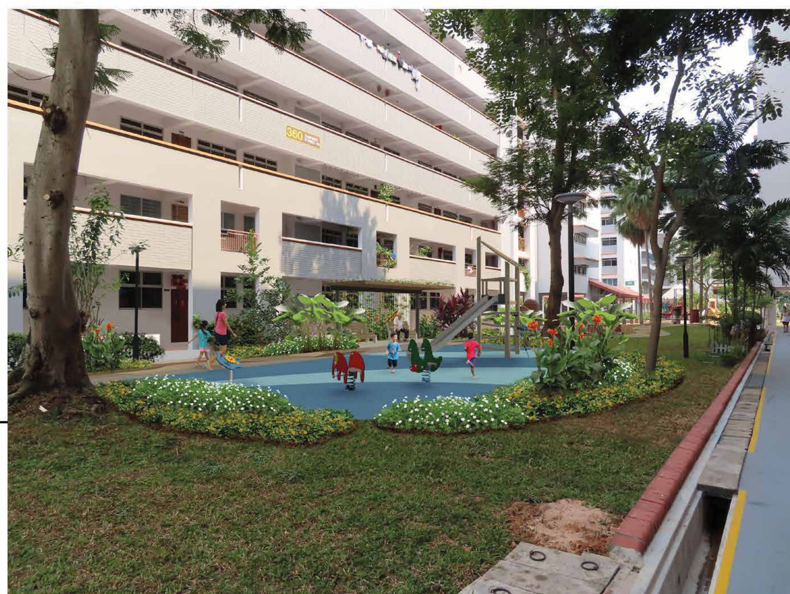
VIEW OF INTER-PRECINCT CONNECTOR BETWEEN BLKS 359 & 360 MODIFICATION TO EXISTING PLAYGROUND MAY BE REQUIRED
