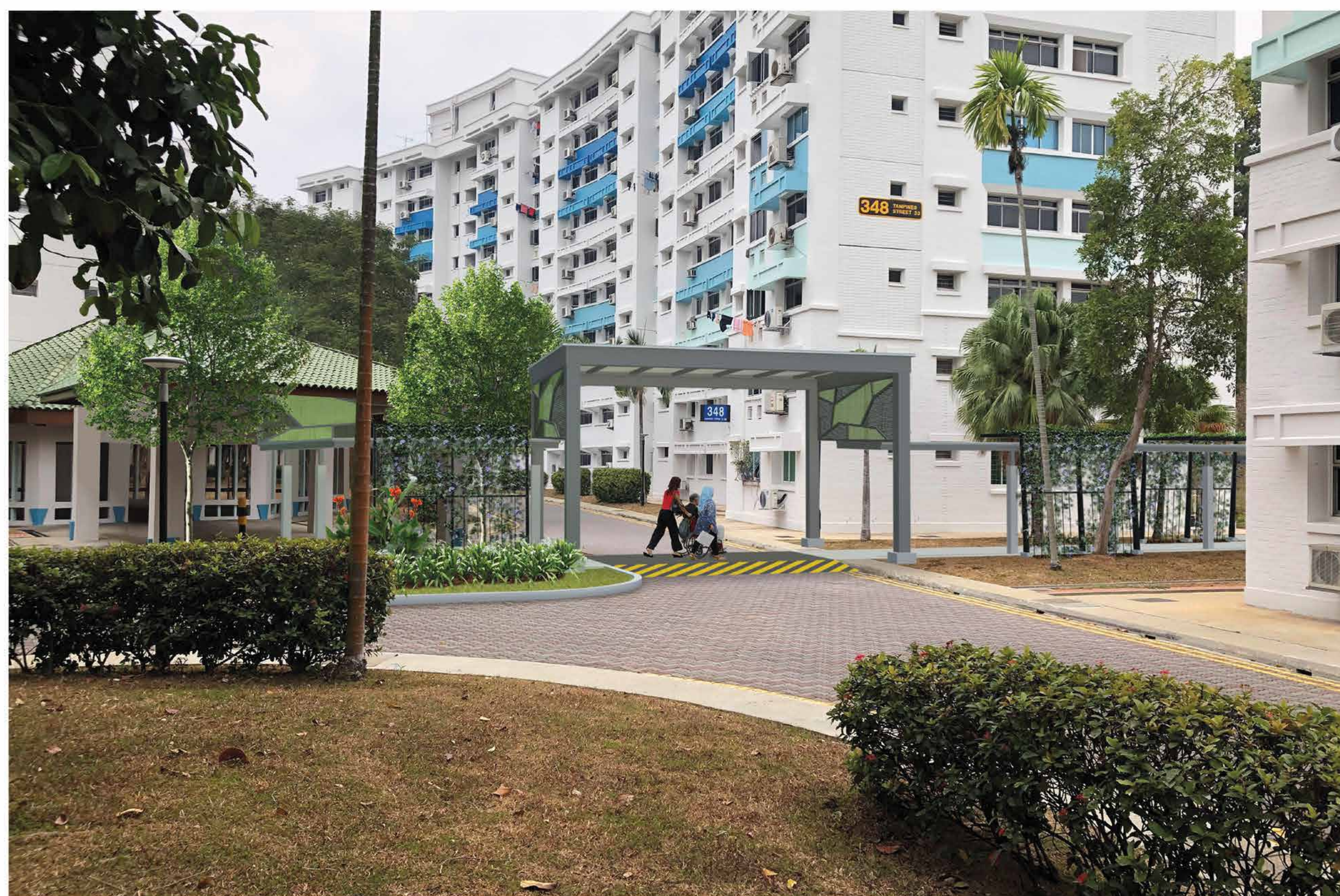
VIEW OF LOW LINKWAY & HIGH LINK FROM BLKS 347 & 348 TO DROP-OFF PORCH AT PRECINCT PAVILION
